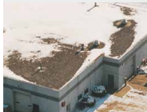
First Firestone EPDM roof installed in 1980 in Wisconsin, USA, still performing well today.
